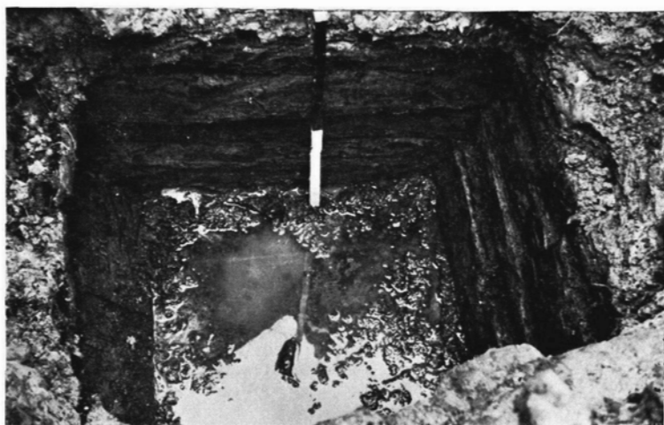
A. Timber lining at bottom of Roman well.
